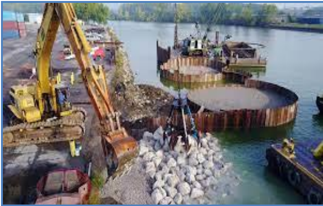
The construction phase
