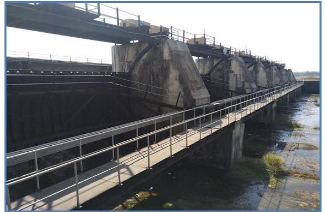
The Darna Dam site
