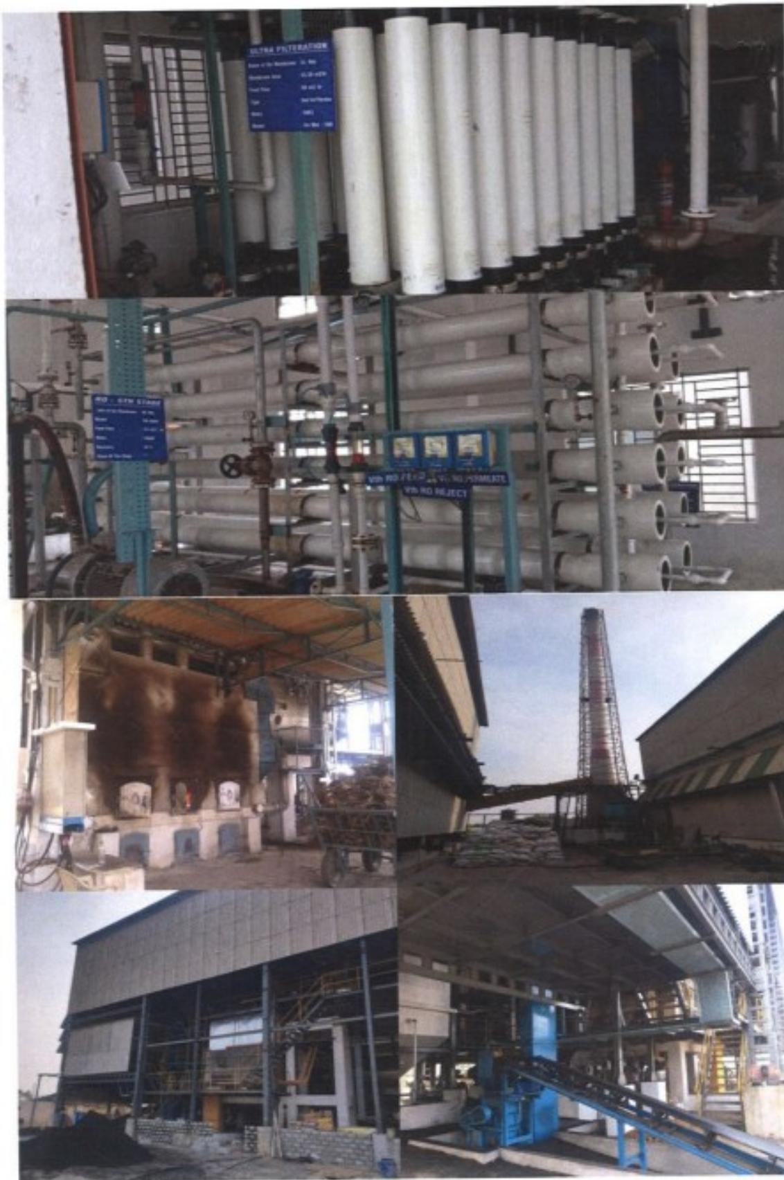
Ultrafiltration, Additional Stage RO and Boilers at Kasipalayam CETP
