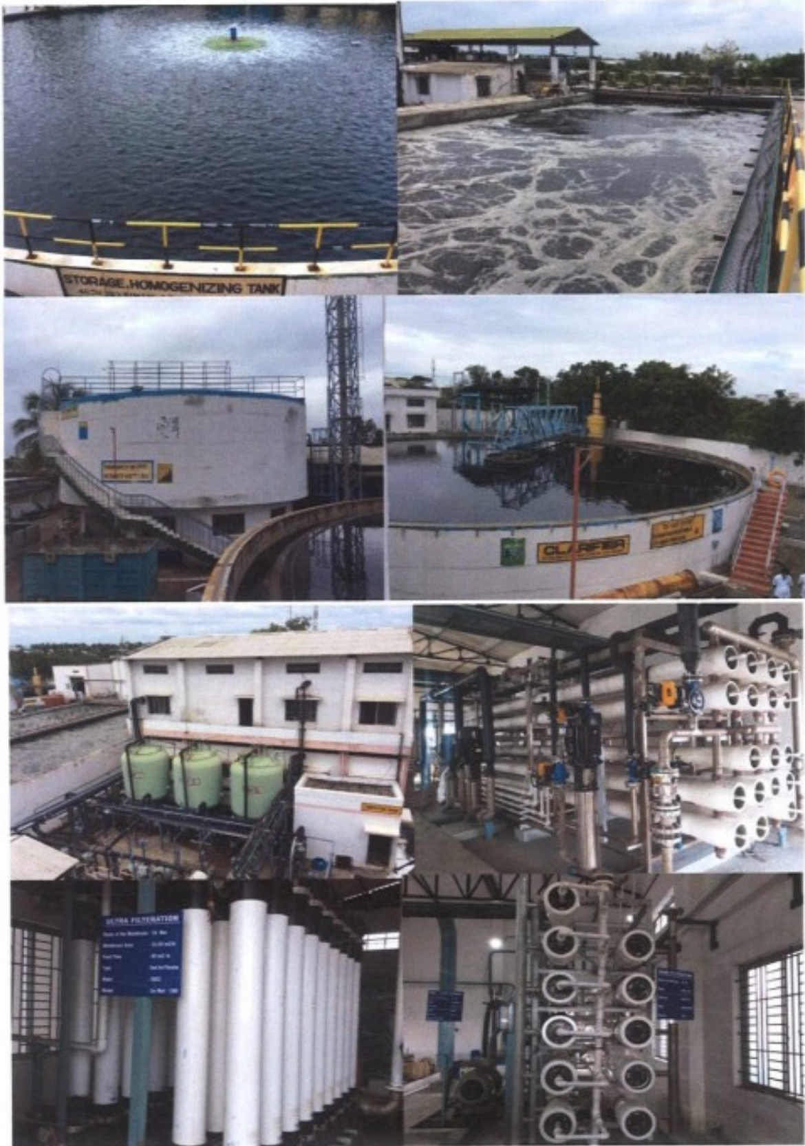
Effluent Treatment units of Kasipalayam CETP
