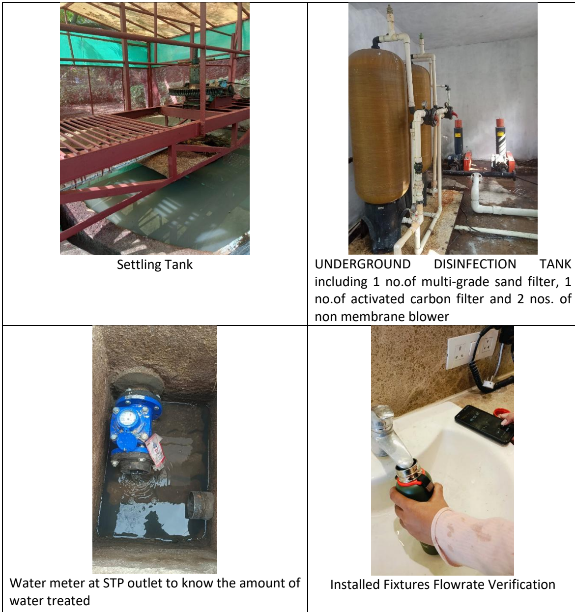
Figure 11.14: Site Survey - Club Mahindra Kensville
